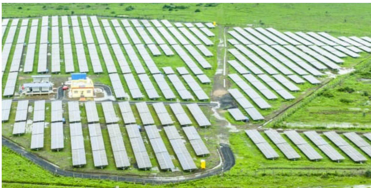
Solar Plant at GAIL Vijaipur
